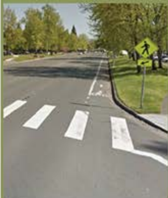
CONTINENTAL CROSSWALKS / CRUCE PEATONAL CONTINENTAL
