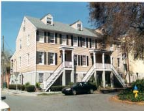
Fig. 4.3.2 This tri-plex in Savannah, Georgia, with its individual entries right on the street integrates very well with surrounding single-family homes.
