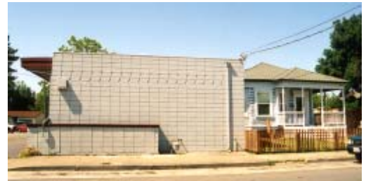
Fig. 4.3.4 This repair garage on Sebastopol Avenue is a particularly bad fit with the neighboring homes. The front setback, the blank wall at the front elevation, the concrete block, and the flat roof/parapet are all out of character with the existing single family homes.
